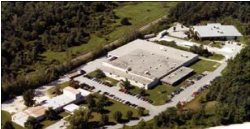
Harbour Industries Facility in Shelburne, Vermont.
