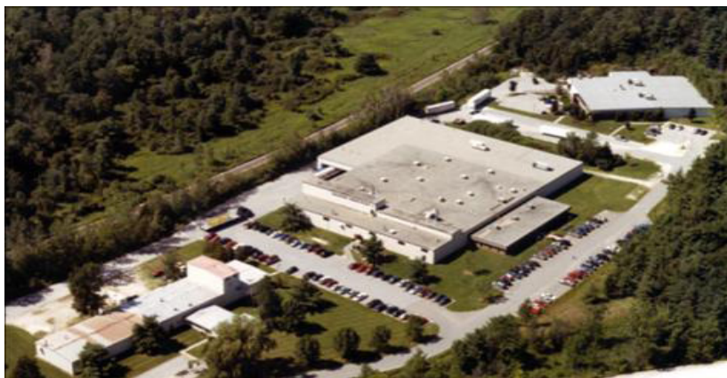
Harbour Industries' Facility in Shelburne, Vermont
